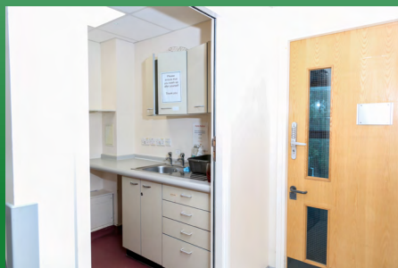
The parent kitchen before renovation began.
